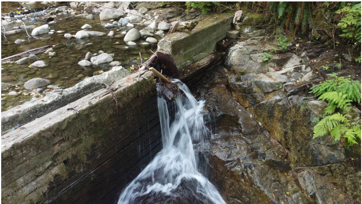
Photo 4 Control Structure on left side, view 1.
