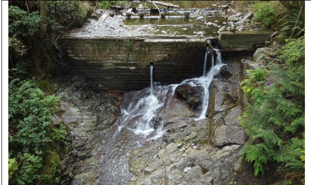
Photo No. 1 Date: 19 September 2023 Looking Towards: West Location: Mackie Road Dam Description: Looking at Mackie Road Dam during the low flow period.
