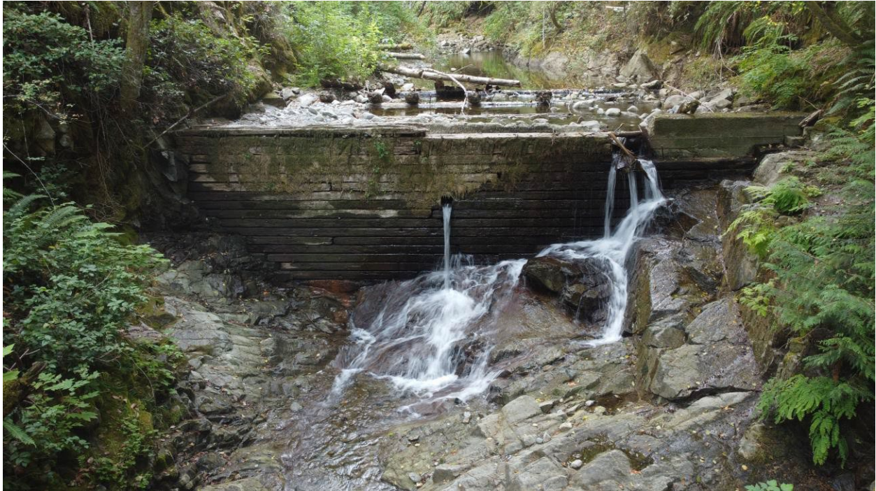
Photo 1 Downstream face of dam, looking southwest.
