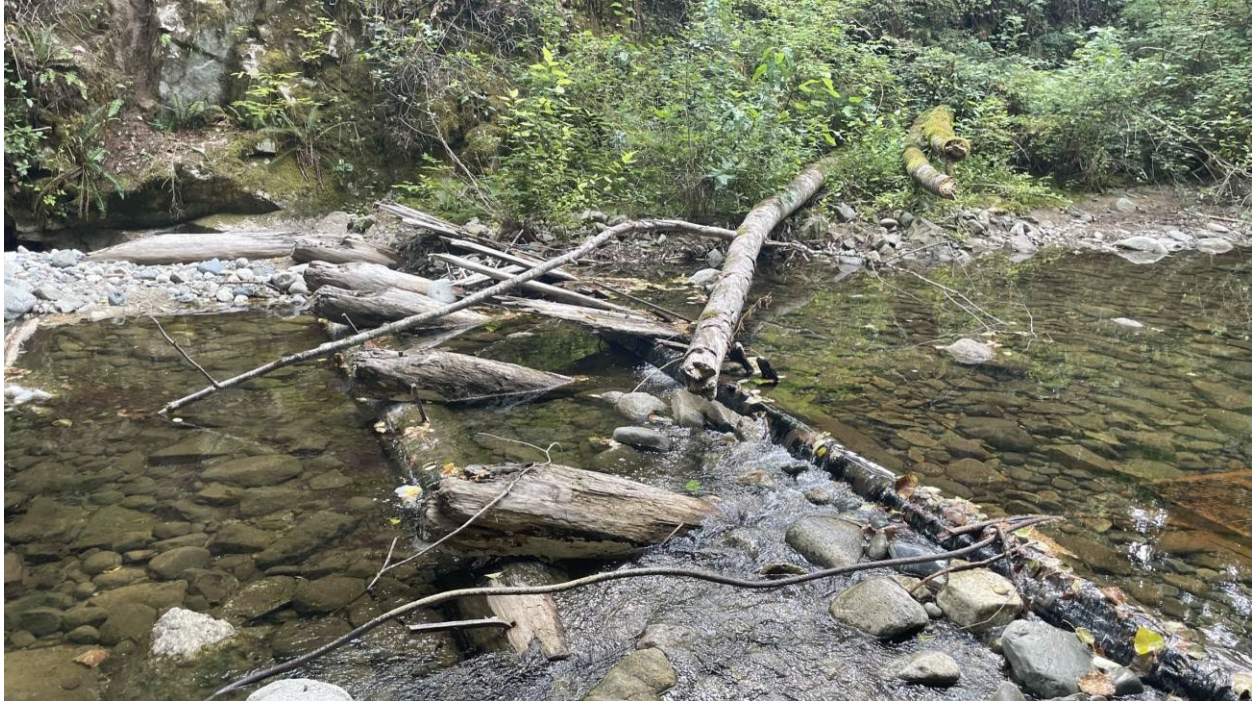
Photo 8 Vegetation built up on remnants of wooden flashboards on right side of upstream channel & miscellaneous debris.
