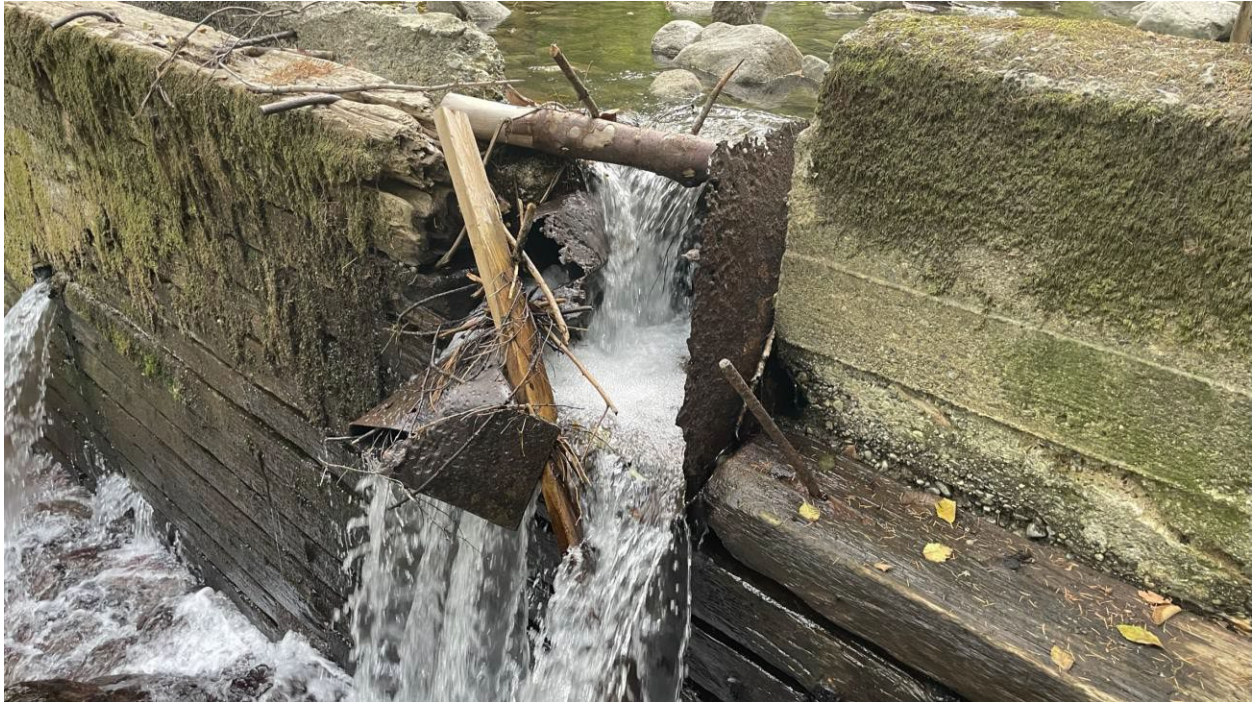
Photo 5 Control Structure on left side, view 2.
